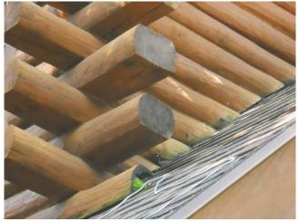
does not run directly against the logs in this area. In a situation like this, we have replaced the rotted logs and cut in the flashing so that this new flashing detail could
