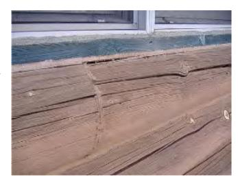
moisture gradients between the inner and the outer parts of the logs causes these checks.
