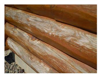
breathe. Modern log home finishes not only seal water, but also allow for the logs to breathe. Many times when stains are over-applied or get built up, we see issues with rotting logs. This is why log home finishes have a two-fold purpose: seal up the logs while still allowing them to breathe.
