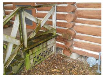
continually getting wet causes them to rot. Rotten logs can be very expensive to replace especially if they are the bottom logs in the wall.
