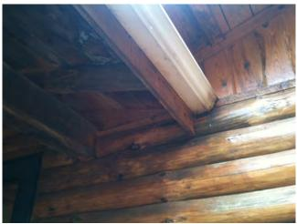
wall. <u>Click here</u> to see a diagram of the proper way to flash a deck to a log wall. Certainly doing the flashing correctly the first time is always the best but this type of deck flashing can also be retrofitted to an existing situation.
